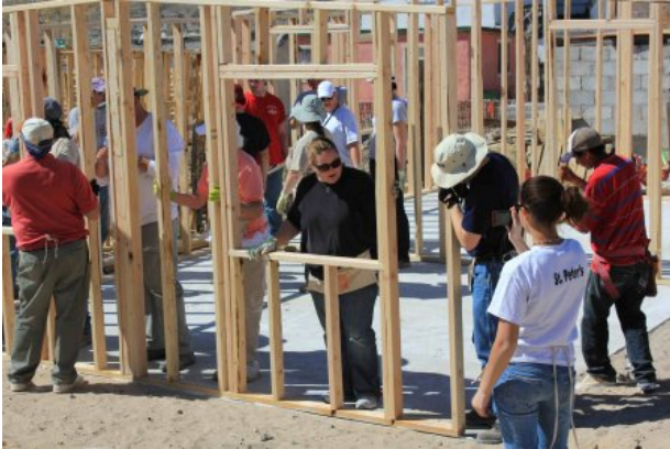
Putting up the frame
