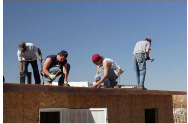
Myles and Theo install roofing.
