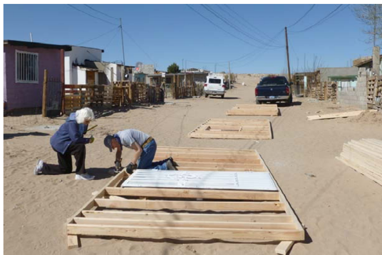
Framing the walls
