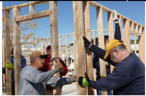
Putting up the frames
