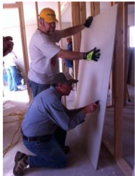
Cutting the sheet rock
