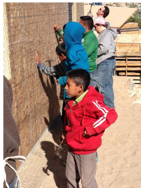
The family helps nail up the chicken wire.
