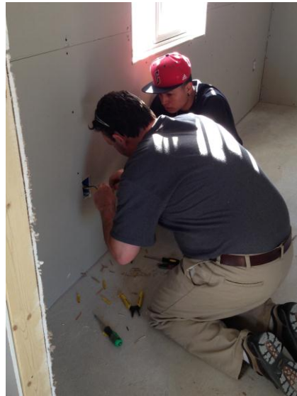
Finishing up the wiring
