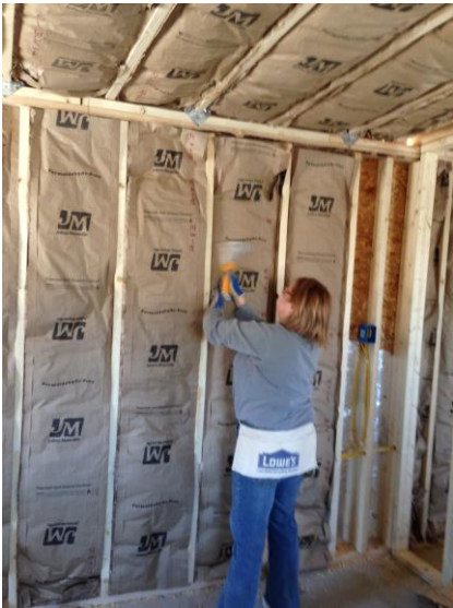
Beth nailing up the insulation
