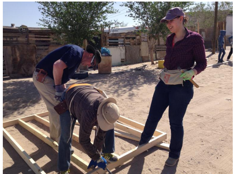
Chandler, Natalie and Beth hammering the wall studs.
